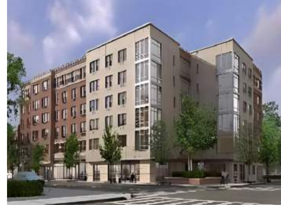
DASNY New Life Recovery Center Bronx, NY HPD Bronx Lebanon Hospital
