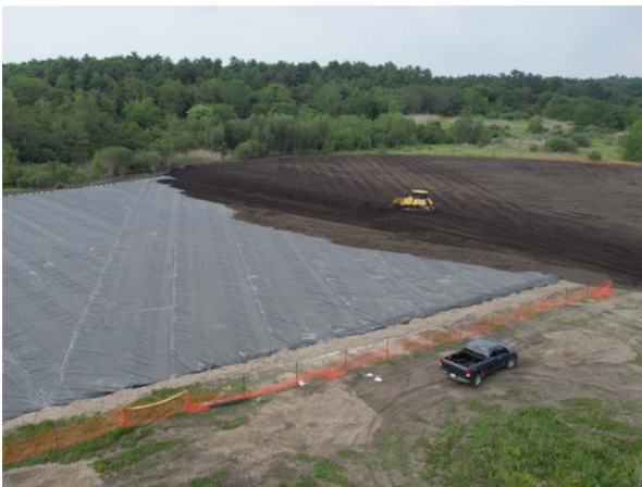
Figure 2.2. Remediation work underway at the Carver Industrial Park.
